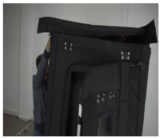
**Please note:** With two people after you place the roof panel on the frame – one person should help from the inside by pushing the panel upwards and disconnecting from Velcro and the other person would align the roof from the outside. Once the roof is squared on the top the person on the inside would unfold and attach the interior flap. To finish up seal the roof with the exterior flaps.
