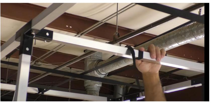
When the frame is set up, hang the 3 acoustic blankets on the frame with velcro straps – we recommend installing them on the inside
