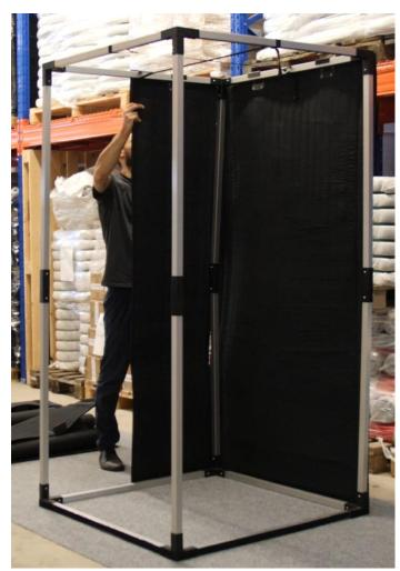
After all the wall panels are instaled, put up the roof panel on top.
